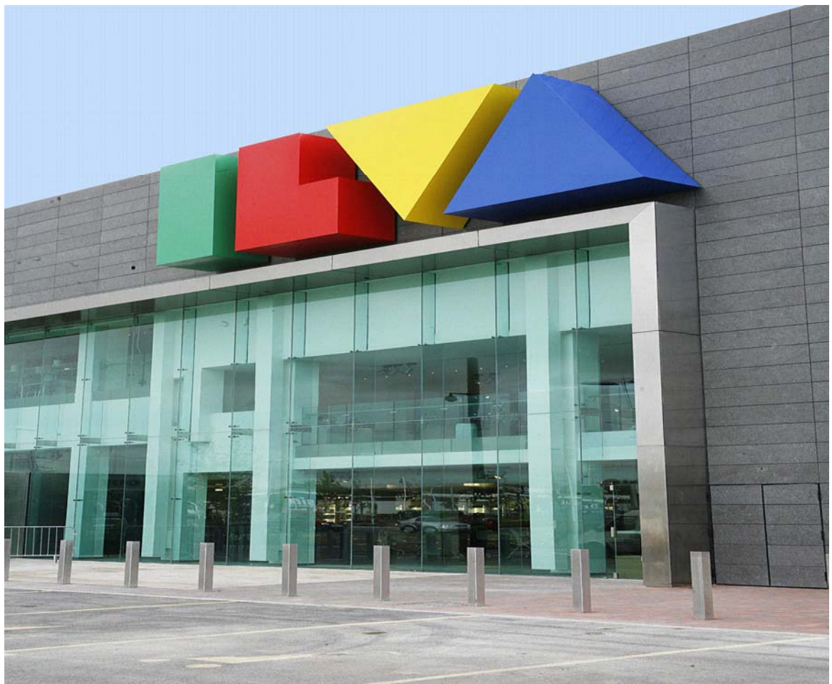
Figure 3: ILVA store exterior
